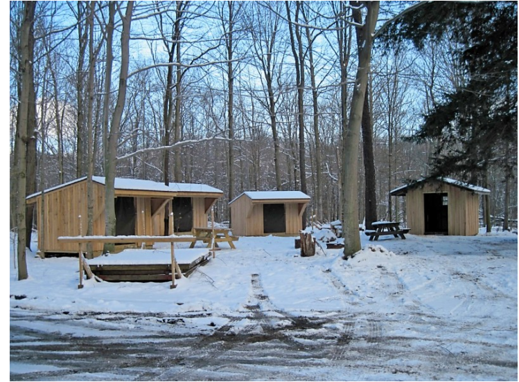
Three of the six new lean-to's, plus the rebuilt hut
