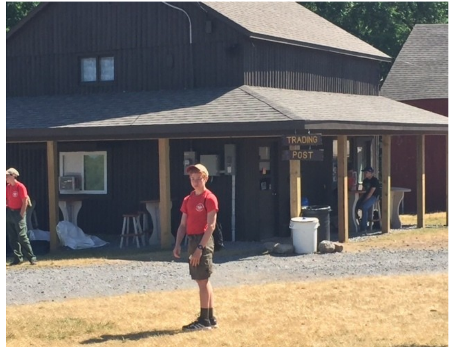
This pictures shows the porch that was added to the Trading Post at Camp Dittmer. The project was funded by Ashokwahta Lodge.
